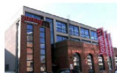
4. Kesselhaus / Fitnessstudio Bleyle LOFT
